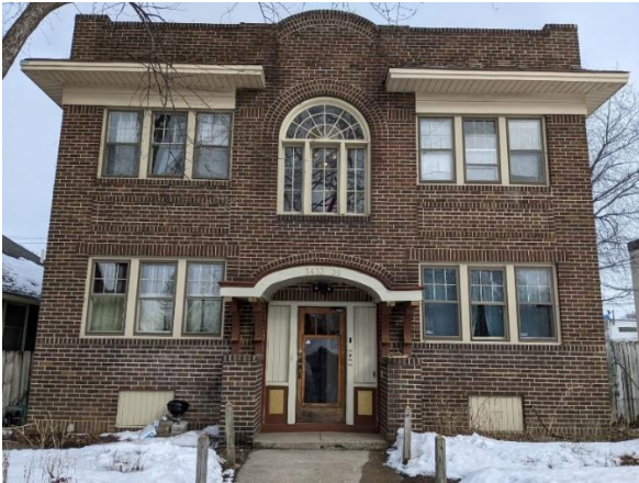
Figure 6. Site 5, “Quanta Multifamily #3,” five-plex multifamily with 30 windows, window age estimated 60–120 years. Contractor-installed product: exterior Low-E storm windows.
