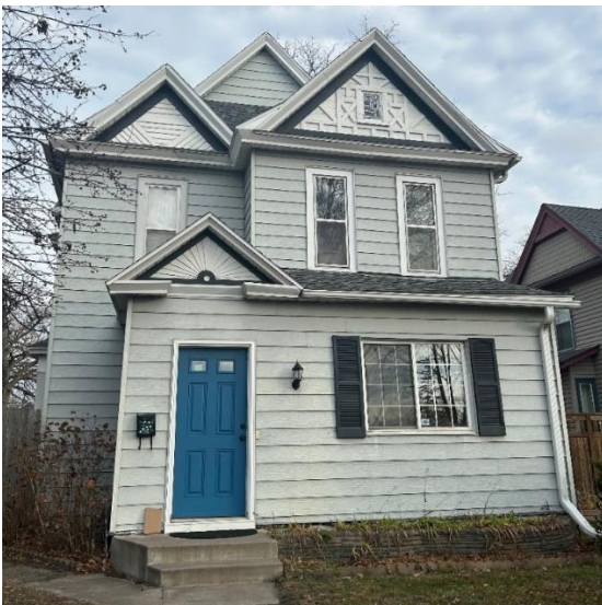
Figure 2. Site 1, “Indow Single-Family,” single-family unit with 25 windows, window age estimated 60–120 years. Homeowner-installed product: interior non-Low-E storm window inserts.
