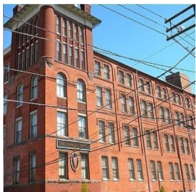
1892 Umbrella Works, Lancaster PA - adaptive reuse to apartments, interior low-e panels.
