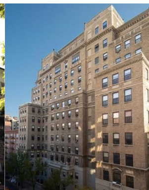
1929 French Apartments, New York City, NY - interior operable low-e panels. Photos courtesy of Quanta Panel
