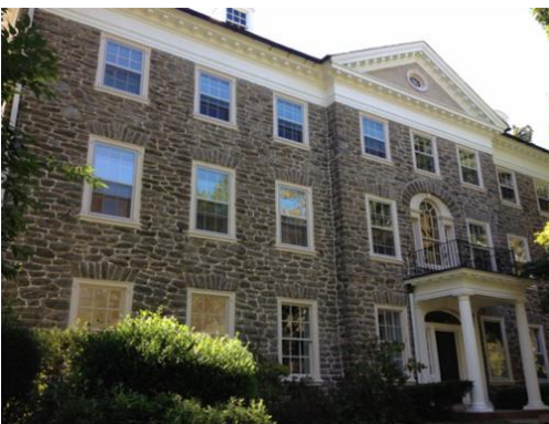
Wissahickon Avenue Apartments, Chestnut Hill, PA - exterior low-e storm windows.
