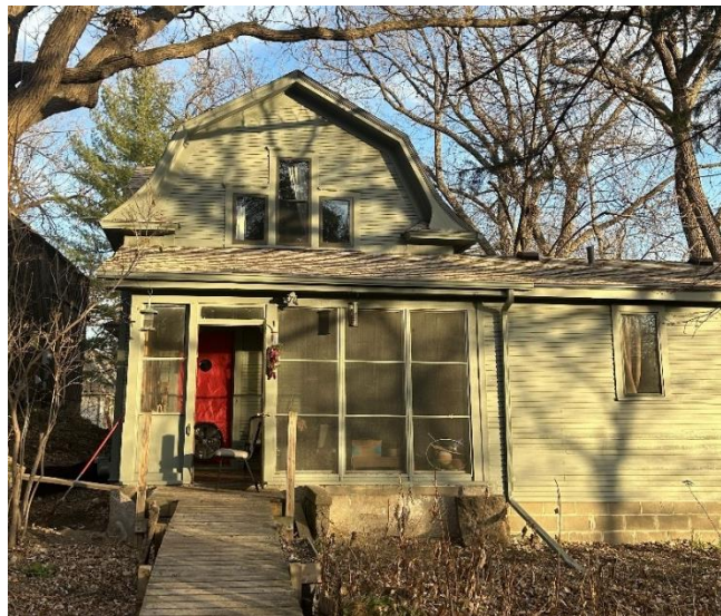
Figure 3. Site 2, “Mon-Ray Single Family,” single-family unit with 31 windows, window age estimated 60–120 years. Homeowner-installed product: exterior non-Low-E storm windows.
