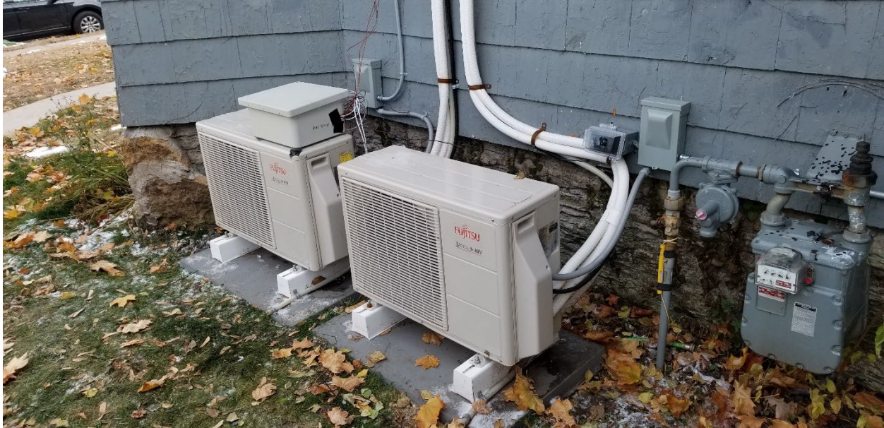
Figure 8. Outdoor unit installation at MF_01
