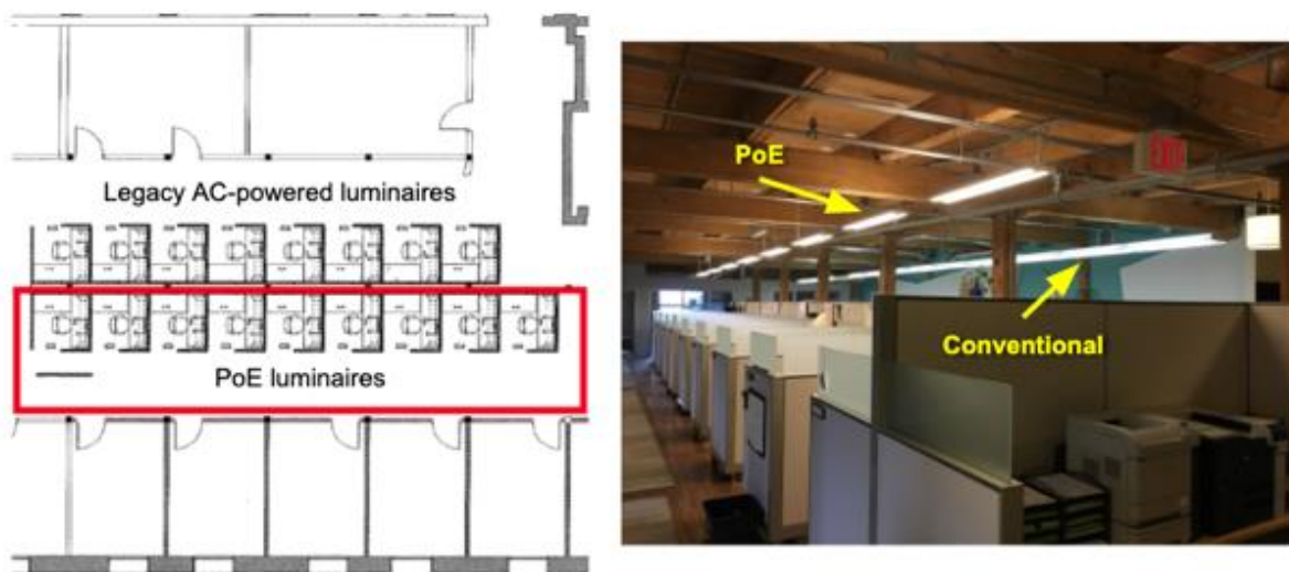
Figure 12. Floor Plan and Photo of the Networked (PoE) and Non-Networked Legacy Lighting Systems over the Rows of Office Cubicles.
