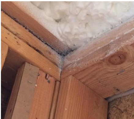
Corner of wall assembly
